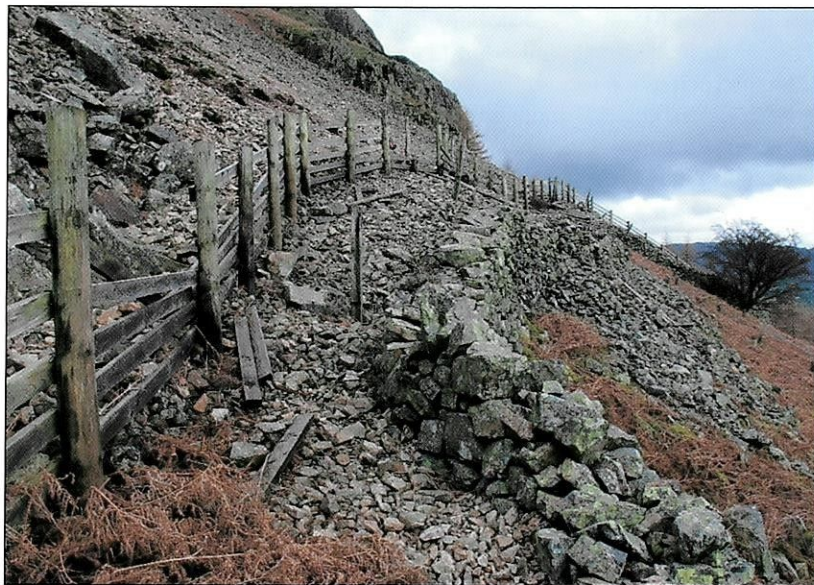
Figure 1. Wall above the Old Dungeon Ghyll Hotel in Great Langdale overtopped by downslope movement of talus.
