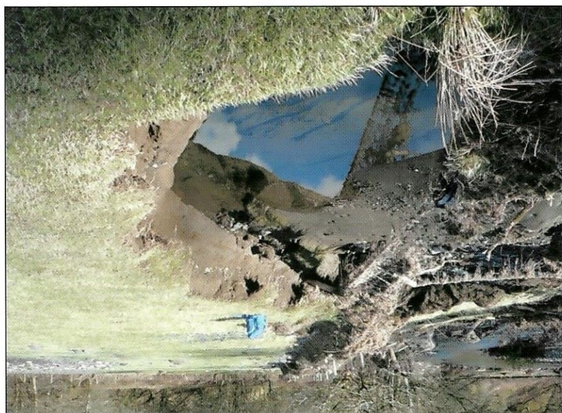
River Greta Bank erosion occurred in a number of places removing sections of the old railway line track.
