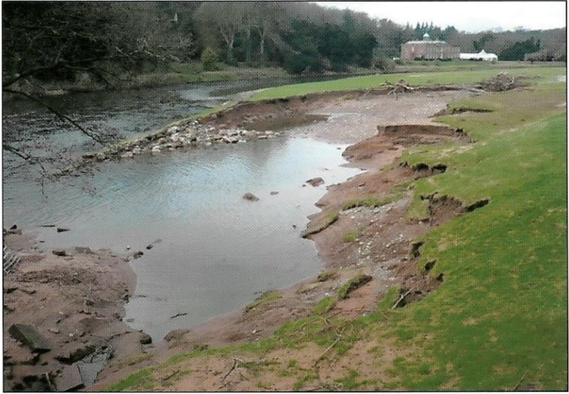
River Eden, Warwick Bridge
