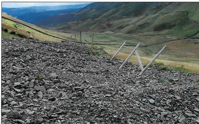
Figure 8. The debris of Fan 11 is level with the top of the wall and has spilt over into the enclosure. It has also disturbed the fence that was built to maintain the boundary and prevent sheep from jumping into the enclosure.
