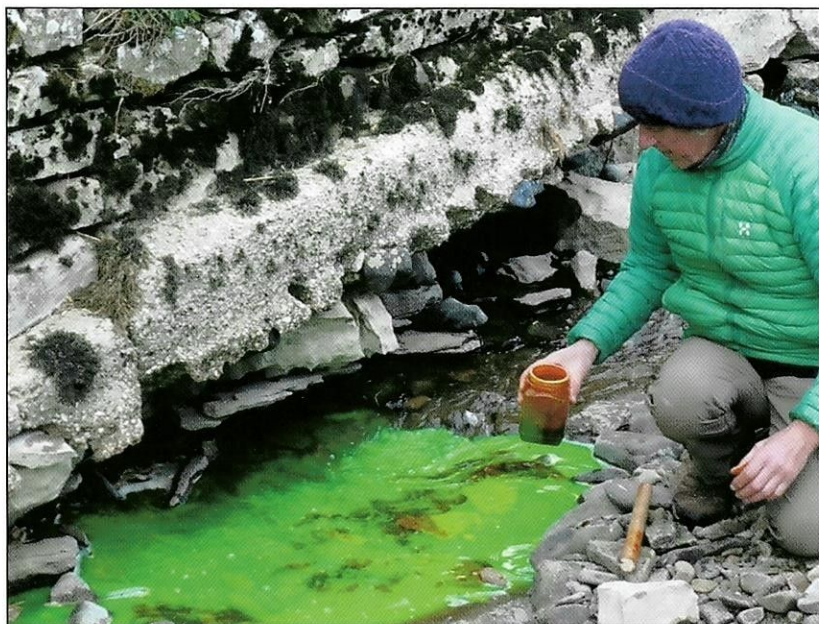
Figure 28. Sodium Fluorescein Dye Testing in sinkhole below NE corner Tarn Gill Bridge.
