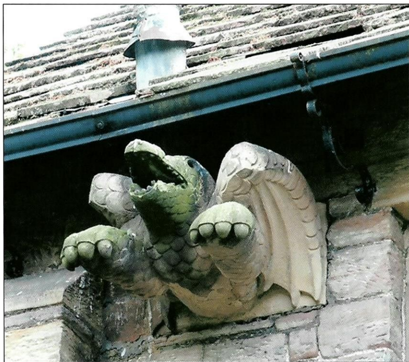
Figure 8. The 'dragon' hiding the exhaust from the (original) heating boiler.
